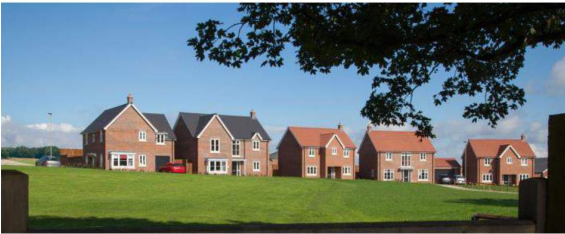
The photos here show some constructed dwellings from Phase 1.
